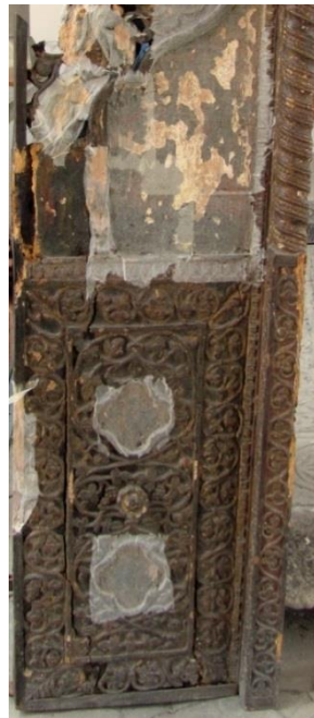
7. Losses of wooden material on the extremities; detail
