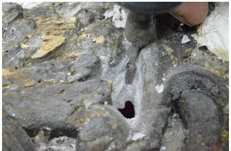
14. Detail; removal of the epoxy stucco excess on the sculpted decoration level
