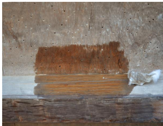
7. Detail; cleaning of the backside
