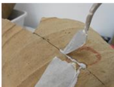
34. 35. 36. Cracks puttying
