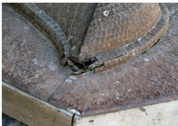
3. Wooden material and missing nails
