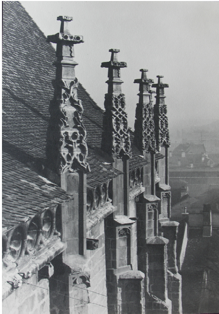
Fig. 14. Artificial stone replicas of the choir pinnacles (photo, 1937)
