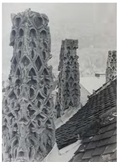
Fig. 12. Deteriorated pinnacles on the polygonal termination of the choir (photo, 1935)
