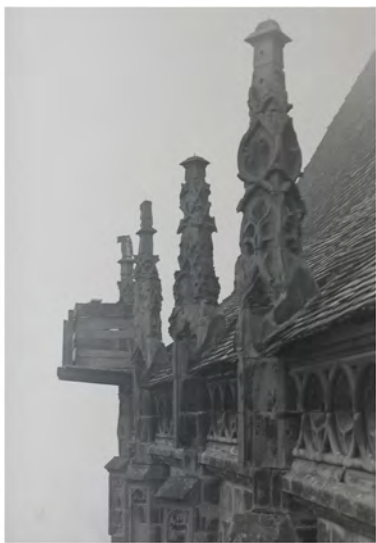
Fig. 11. Deteriorated pinnacles on the Northern side of the choir (photo, 1935)
