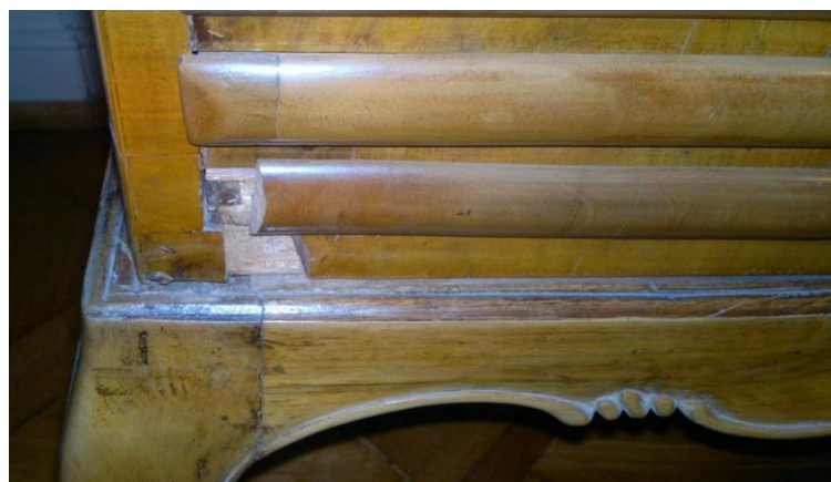
6. Detail; losses of wooden material
