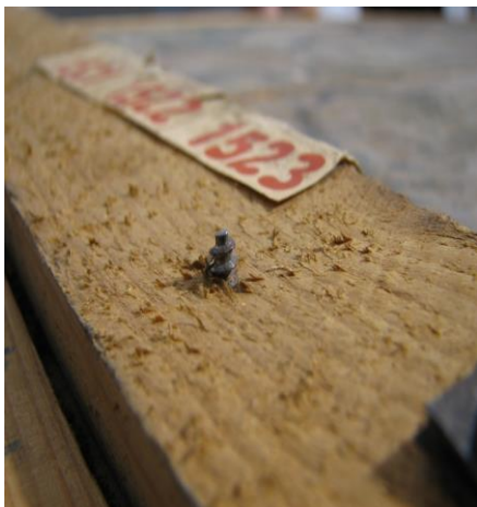
5. Detail; added metallic elements
