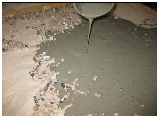
11 a, b. The aspect of the surface after the first layer of fine roman cement was casted
