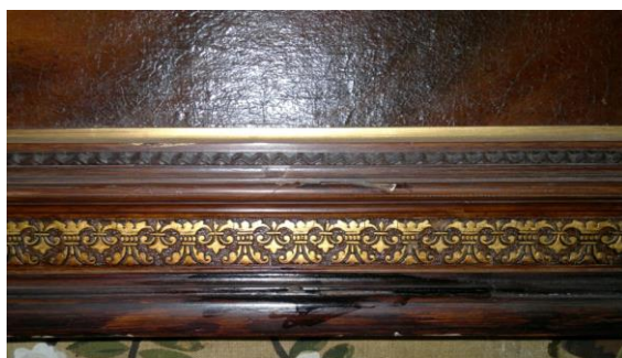
12. Detail; improper chromatic integration
